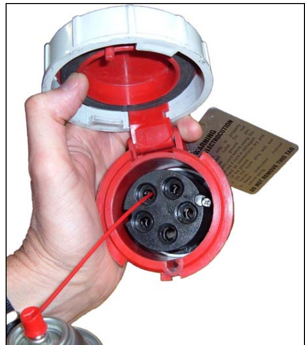
Figure 10: Lubricate the receptacle.
