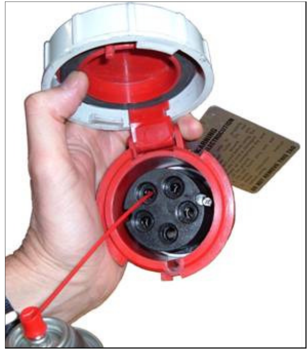
Figure 14: Lubricate the receptacle.
