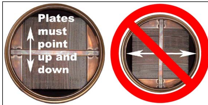
Figure 6: MDPF plates must point up and down for horizontal installations.
